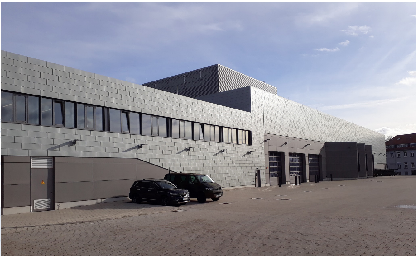
The new multi-purpose building, completed in January 2021, provides 5,000 square meters of efficient workspace.
